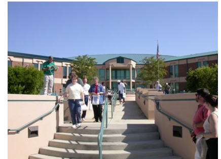
The Frank C. Amerson Jr. Water Treatment Facility in Macon, GA.
